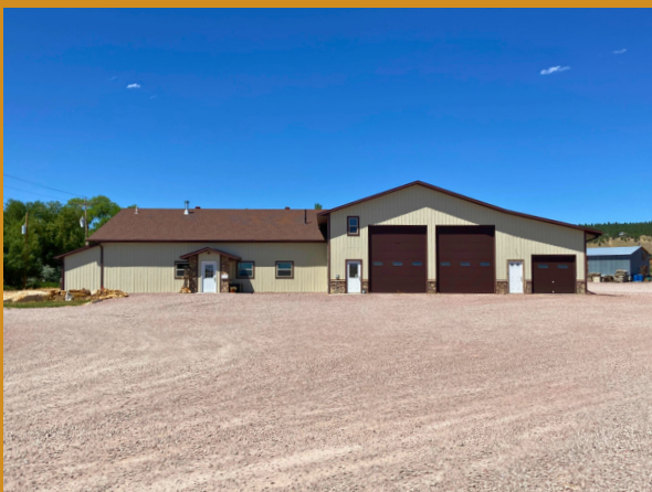
“The Plumbing Shop” before renovations began.
