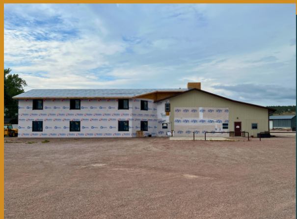
The building as it looks currently. It’s beginning to look like a church!
