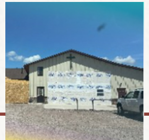
Newcastle, WY New Classrooms
